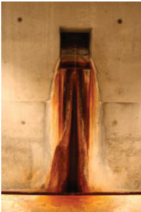
Figure 8. Therme Vals, interior space (Author).
